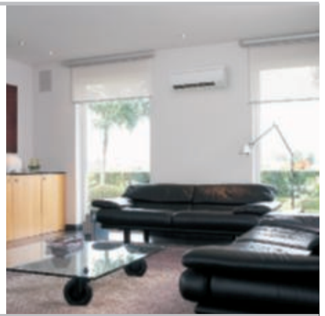
Wall mounted unit >
